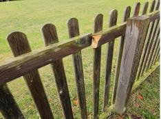
The fencing is in very poor condition with one broken top rail and broken or missing fence slats, there are 8 loose or rotten posts and the second leaf gate at the entrance is not supported as the post is rotten.
