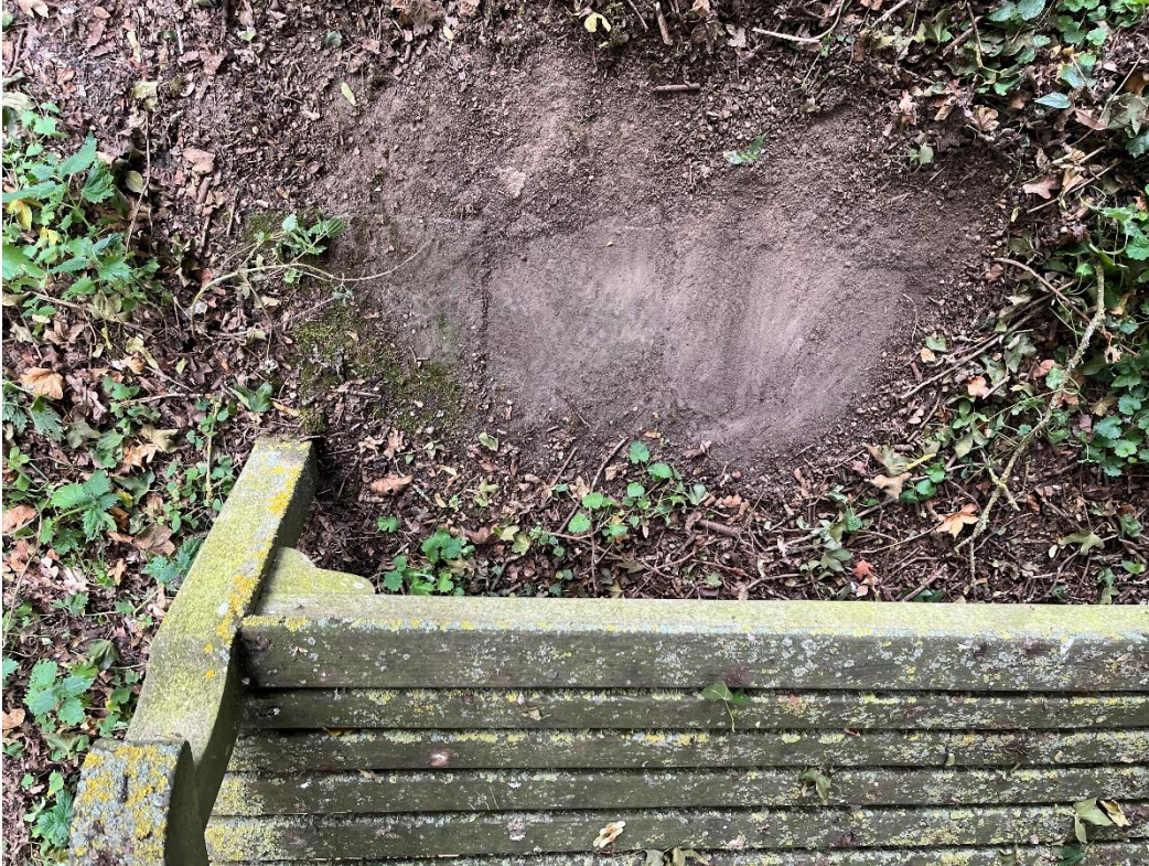
Slabs to front of bench
